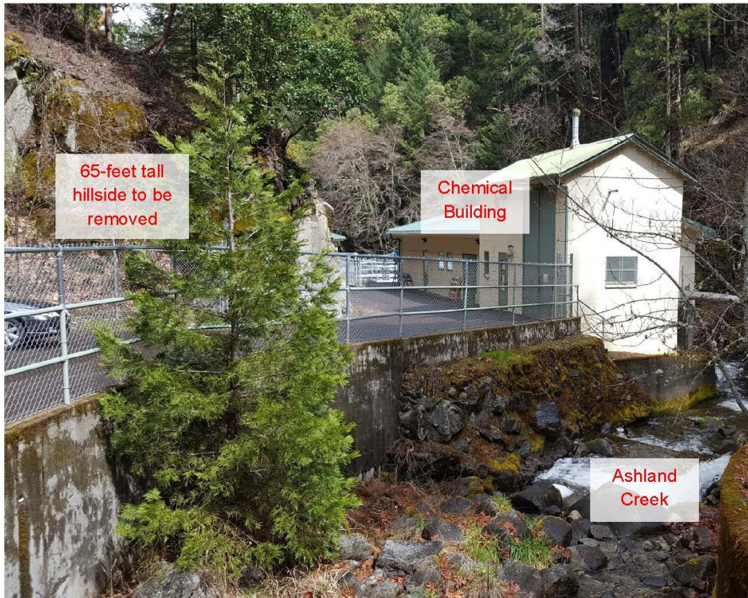
Figure 3. Ashland Water Treatment Plant
